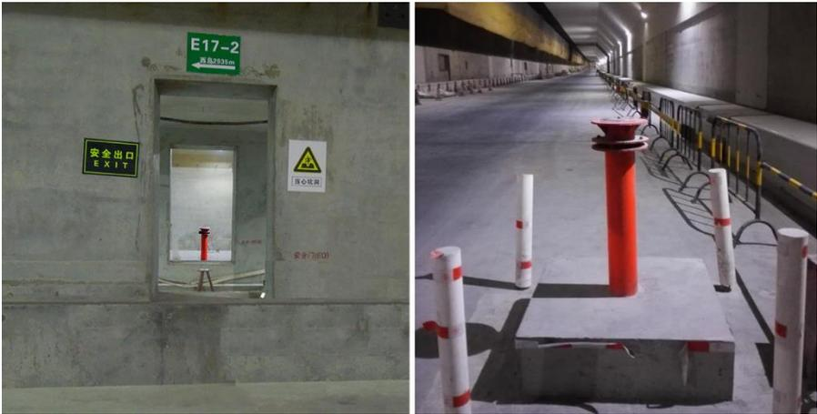
Fig. 6 Inter-visibility between the two bores and steel pillar with forced centering plate
